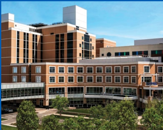
Children's Minnesota Hospital – Minneapolis
